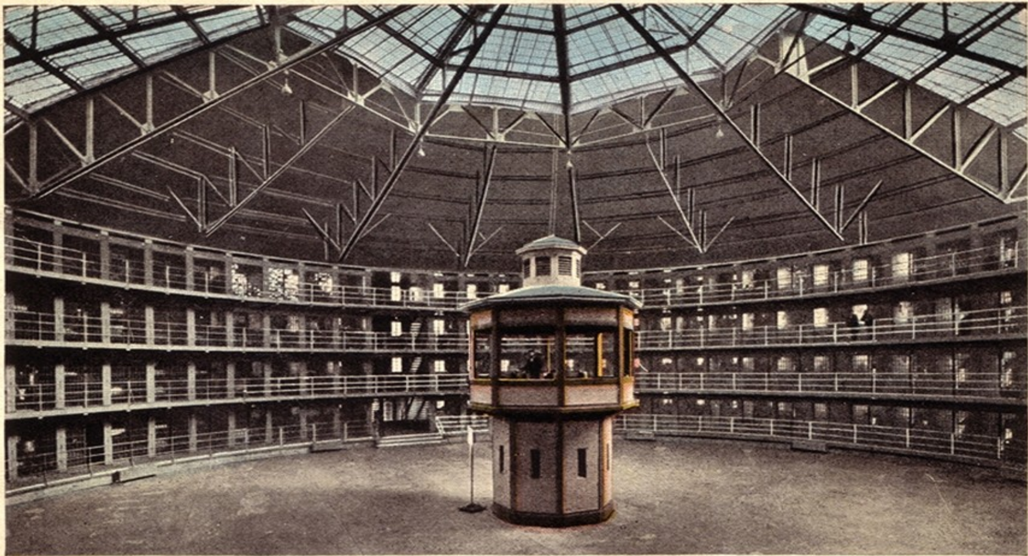
Interior View of Cell House, new Illinois State Penitentiary at Stateville, near Joliet, Ill.—23
